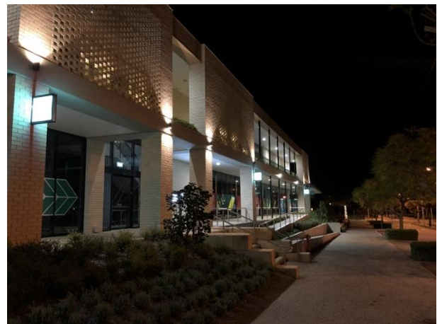
Figure 12 and 13: Example of downward wall lights appropriately selected to minimise light spill at newly constructed Sovereign Place Shopping Centre, noting footpath light spill evident from existing roadway street lighting. Source: Stowe Australia.
