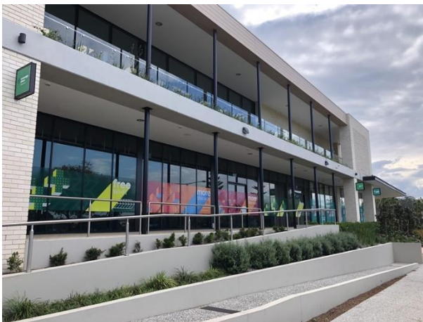
Figure 12 and 13: Example of downward wall lights appropriately selected to minimise light spill at newly constructed Sovereign Place Shopping Centre, noting footpath light spill evident from existing roadway street lighting. Source: Stowe Australia.
